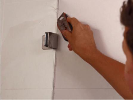
2. Use a cloth soaked in mineral turpentine to clean the newly exposed joint area, ensuring all traces of the silicone has been removed then wipe the area dry.
