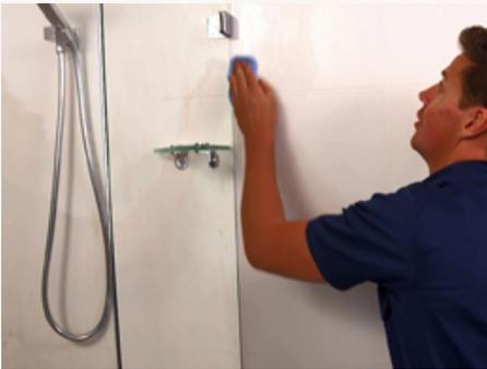
3. Protect the glass screen from silicone with a strip of tape running down its length. Make sure you don't cover the joint though. Do the same for the tile side of the wall.
