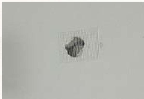
3. Using spatula that's on the lid, gently force some Spakfilla through the holes in the mesh and make sure it completely covers the mesh square around the sides of the hole. For the best seal, use a putty knife or a flexible filling blade to take the Spakfilla across the area in multiple directions. Once the hole is covered, use a single downward stroke to remove any excess product. Allow the product to dry for 30 minutes.
